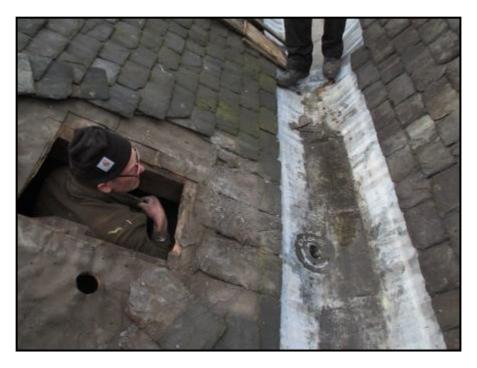
There were a number of leaks from a old lead gutter into a top floor flat in Keir Street. Diagnostic work was done over the winter so that a complete renewal of that main section of leadwork could be planned for the following Spring.
