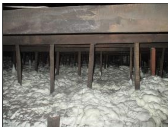
Left - Insulating a fragile ceiling in Lauriston Place where access was very difficult. Foam was pumped from a van in Heriot Place, up the gable.
