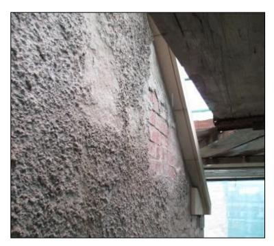
Render on the gable wall at Archibald Place had 'spalled' i.e. lost its adhesion to the underneath surface and then started to drop off, posing a risk to those passing by at ground level.
